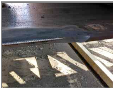
Above - damage to the edge exposing cable
