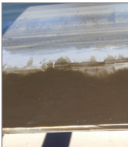
The edge has been rebuilt
