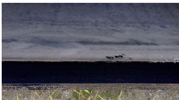
The edge has been resealed
